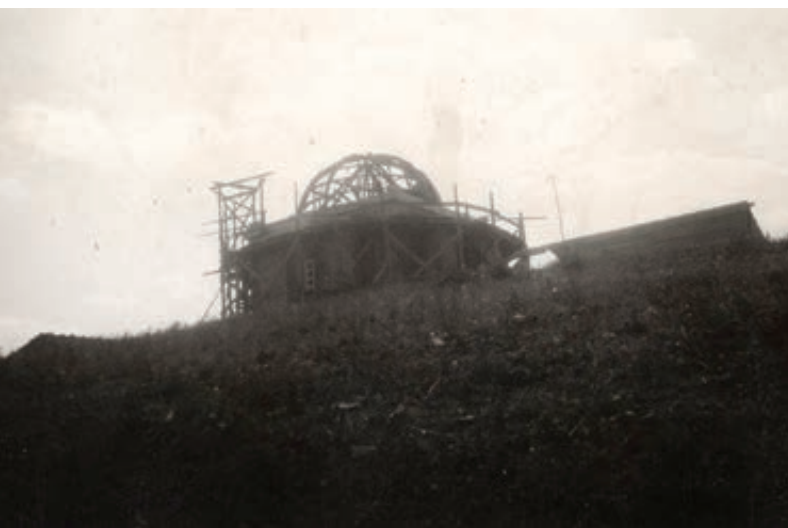
Fig. 10. Church of the Holy Redeemer during construction, 1930 (?) (Photo-Collection of the Meštrović Gallery, Split).
